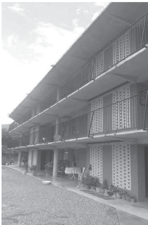
Figure 2: La Habana reconstruction project. Source: The Authors
