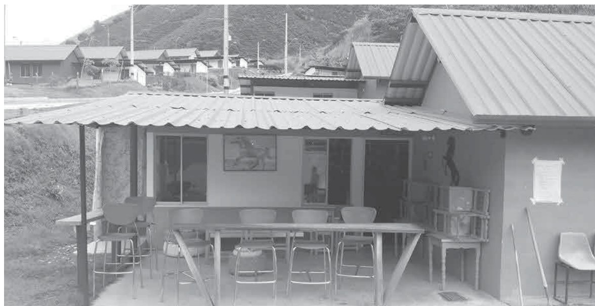
◀ Figure 4 La Pradera reconstruction project. Source: The Authors
